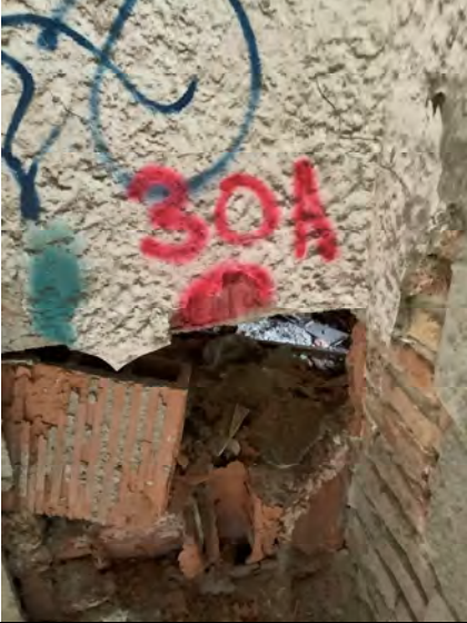
Sample # 30 Plaster - Skim & Base Coat Walls on Brick/Terra Cotta
