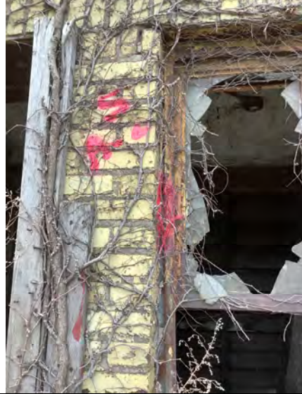
Sample # 5 Exterior Caulk - Around all basement and all other windows
