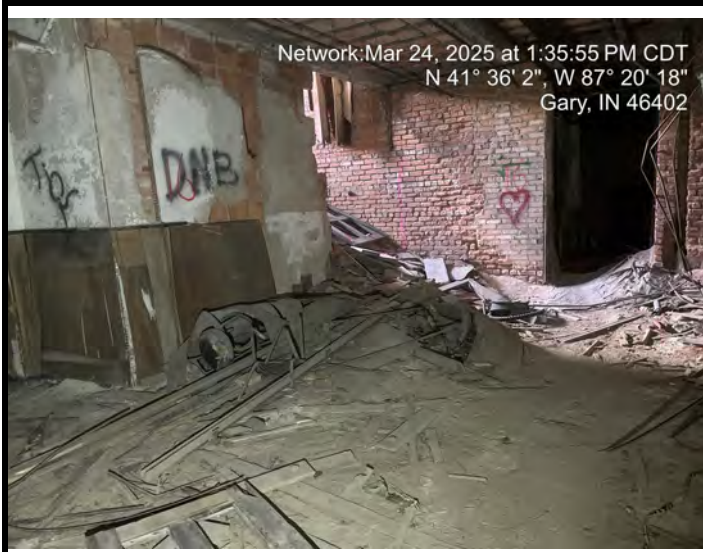
FS-16 Basement Accessible No Issues
