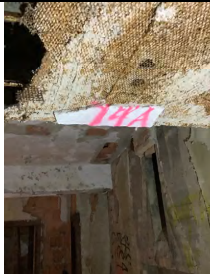
Sample # 14 Plaster - Skim & Base Coat Ceilings on Wire Mesh
