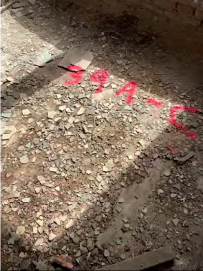
Sample # 39 Flooring - 9X9 Floor Tile with Mastic and Tar Paper- Gray and Green checkerboard Pattern
