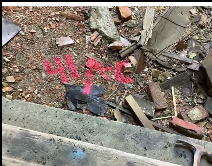
Sample # 41 Roofing Material - Flat Roof Materials
