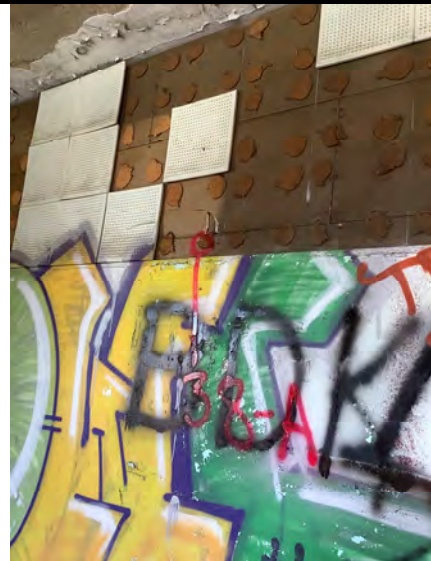
Sample # 38 Ceiling Panel - 2X2, White with Pinholes and Glue Pods
