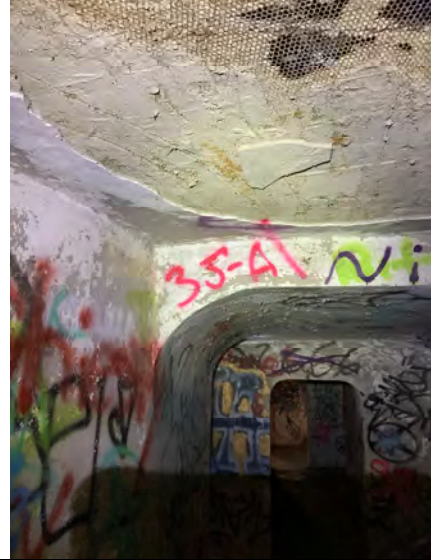
Sample # 35 Plaster - Base Coat Walls on Brick/Terra Cotta ceilings
