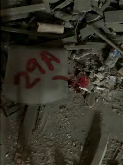
Sample # 29 Plaster - Skim & Base Coat Ceilings on Wire Mesh
