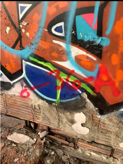
Sample # 36 Plaster - Skim & Base Coat Ceilings on Wire Mesh
