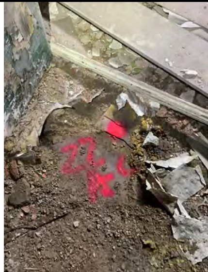
Sample # 22 Flooring - 9X9 Floor Tile with Mastic- Gray
