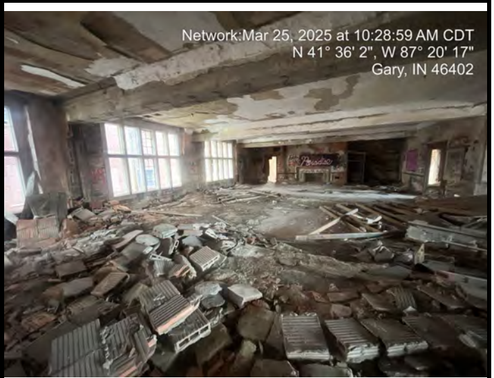
FS-49 Second floor room Accessible No Issues
