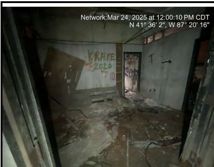
FS-10 Basement classroom Accessible No Issues
