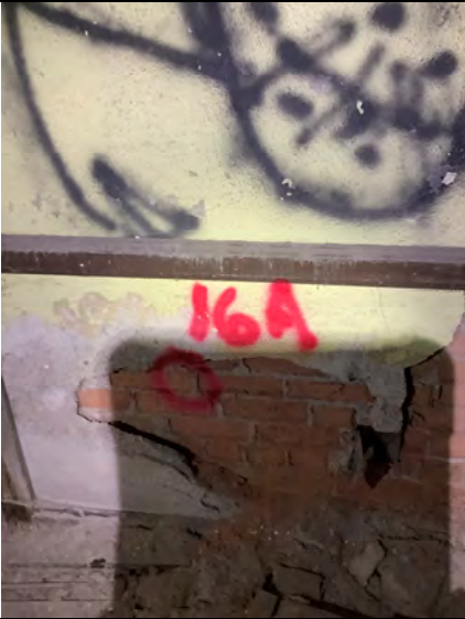
Sample # 16 Plaster - Skim & Base Coat Walls on Brick/Block
