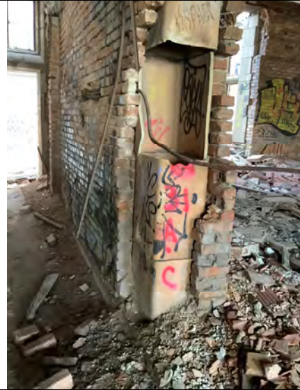
Sample # 31 Chimney Liner - Interior Wall
