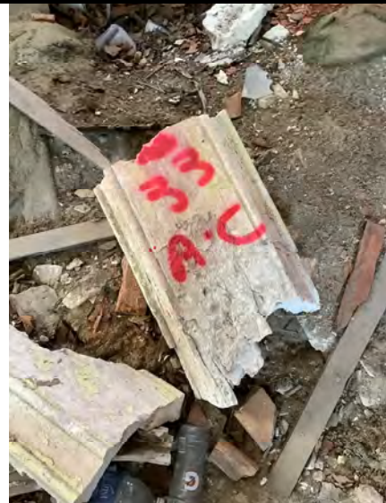
Sample # 33 Plaster - Decorative Moldings
