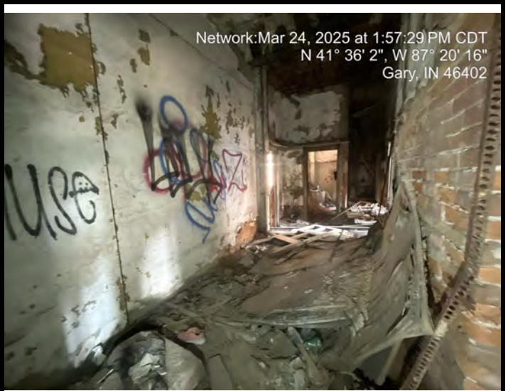
FS-21 Bathroom Accessible No Issues
