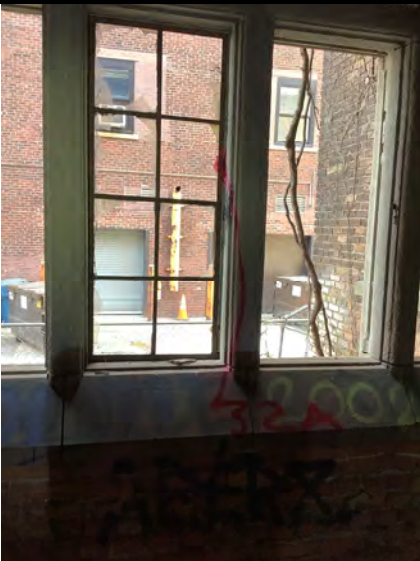
Sample # 32 Window Glaze - Metal Framed Windows
