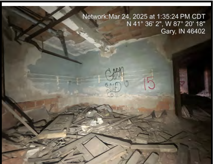
FS-15 Basement coat room Accessible No Issues
