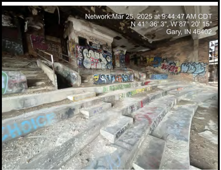
FS-37 Auditorium balcony Accessible No Issues
