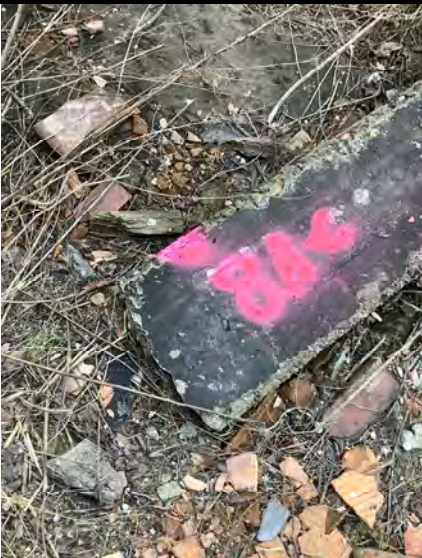
Sample # 8 Waterproofing Sealant - On some concrete blocks
