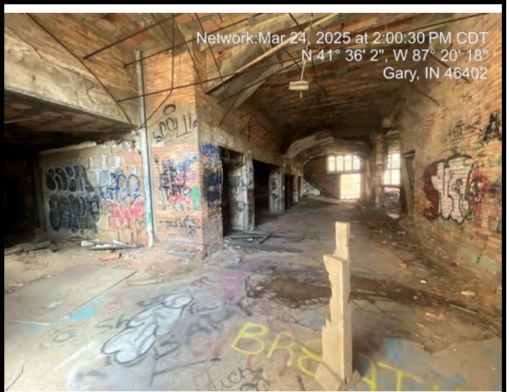
FS-25 Hallway outside auditorium Accessible No Issues
