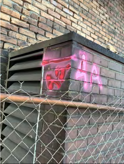
Sample # 4 Exterior Caulk - on Brick Siding air handler building
