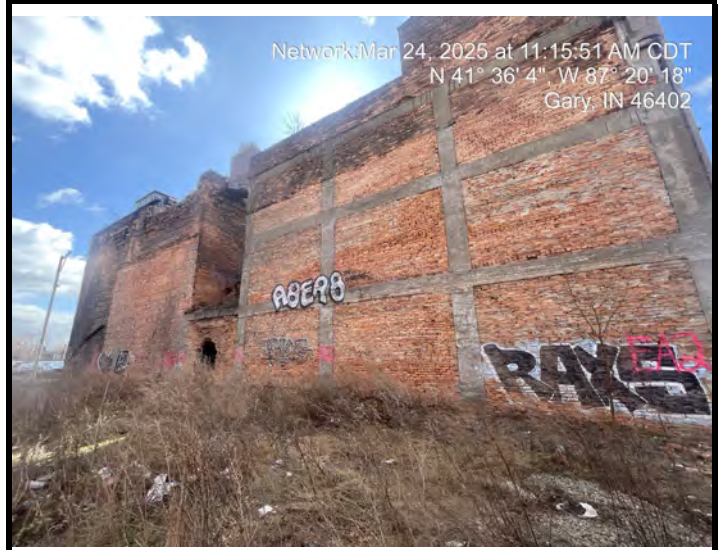
EA-2 Left side of church Accessible No Issues
